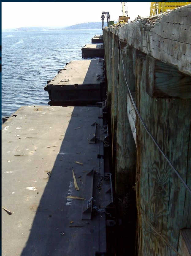
Deterioration of Existing Timber system (East Berth)
